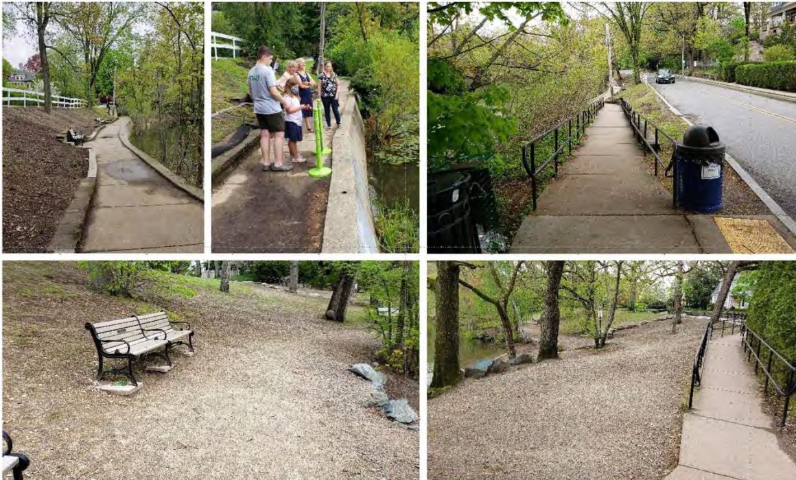
Lack of safety railing, demonstrating fishing with a fishing platform railing, existing ramp, lack of stable ground to access benches, non-contiguous safety railing.
